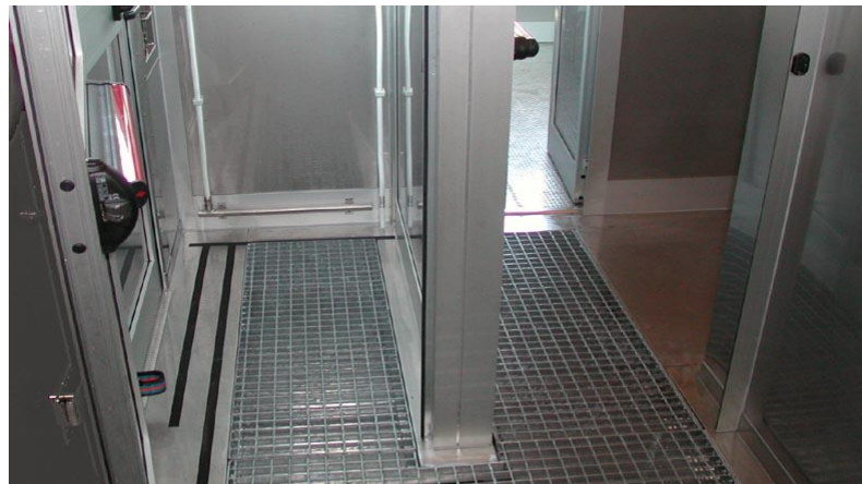
Interior detail of user walkway with tubs protected by grids
